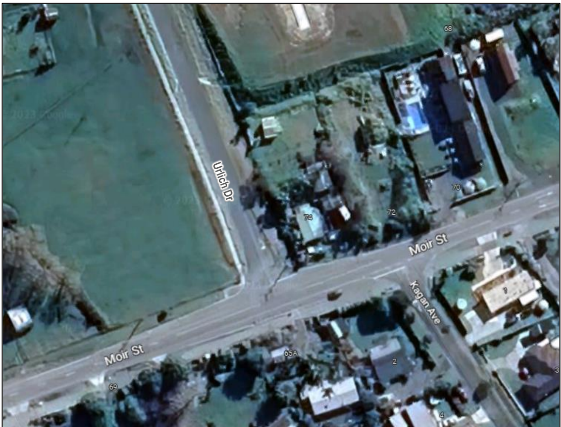
Figure 17: Moir Road and Ulrich Ave Intersection
